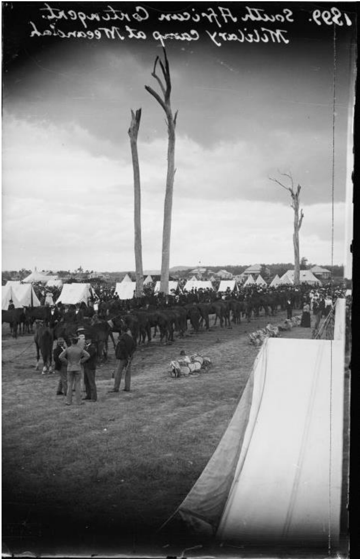
Meerandah camp, looking towards the railway line
